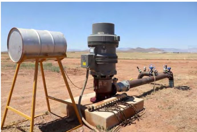
Irrigation well 500' deep, 150 HP, 675 GPM
