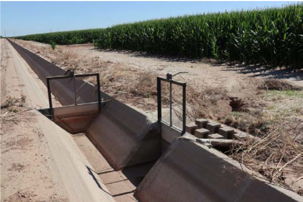
Concrete ditch with typical jack gate turnout
